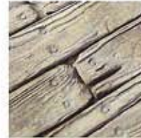
Close-Up of Wood Bridge
